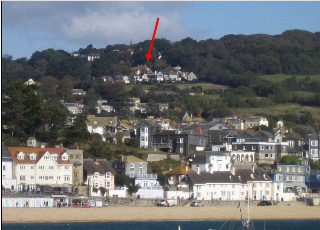
Overton (arrowed) showing its position high “over the town” (2013).
