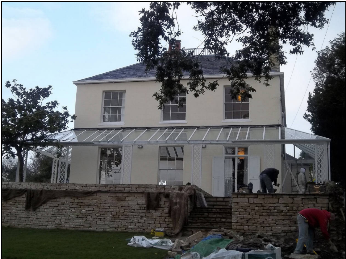
Rose Hill under restoration in 2012 RB
