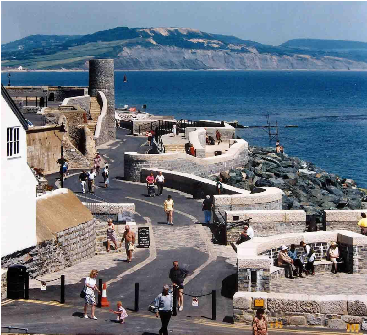
The new sea walls from Bell Cliff, with the new Buddle Bridge (being approached by a person in yellow). The wall tops are coped in Portland Roach to match the top of Cobb Gate Wall, visible in the right foreground. To the left the white wall is the end of Cobb Gate Chip Shop, the building being battered by a storm wave in the Frontispiece, with the eroded top of the old sea wall showing.
