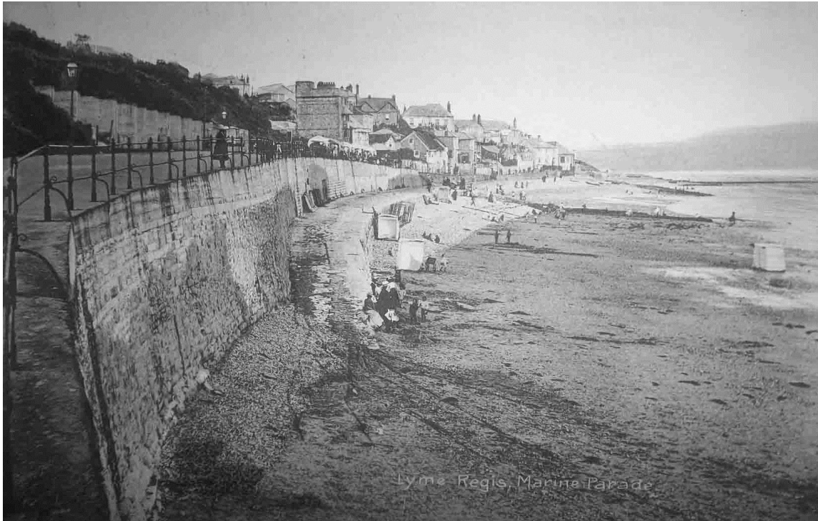
Marine Parade and Cart Road about 1910, showing the ramp to the beach which was replaced in 2005-7. Marine Parade is now railed and surfaced. This section of the Marine Parade wall collapsed in 1939. Concrete buttresses built in 1903 are holding the slope above Marine Parade. De La Beche's Jetty is visible, with the Cart Road going over its head. Development has reached Sundial House, but the Bay Hotel is yet to be built and the Assembly Rooms are still intact. LRM 1989/11-23
