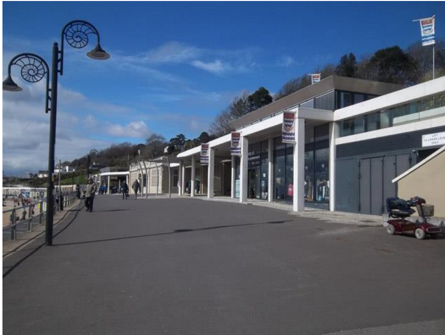
The new restored shelters looking west in 2015, with the Jubilee Pavilion flanked by open shelters in the butress alcoves, in turn flanked by shop units. Plant room and steps on the right, meeting rooms above both shop units.
