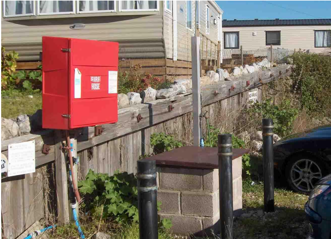
The top of the 1902 Cement Works Sea Wall on Monmouth Beach
