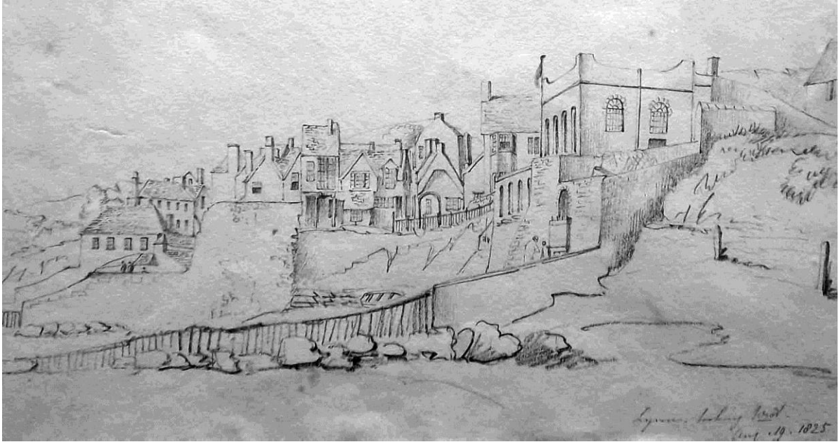
Back Beach to Gun Cliff in 1825, with the Baths, today rebuilt as the Theatre on the right, with Theatre Jetty in the foreground, Gun Cliff and Cobb Gate jetties beyond. The bath chamber openings in the sea wall can be seen, now covered over by a later skin when the sea walls around the embayment were repaired – here, apart from Gun Cliff, they look broken down by the 1824 storm. Guise’s Wall is not shown, as it was lost 30 years before this sketch. Guildhall Cottage is on the brink and looks precarious, although there is a post and railing fence along the walk up to the Baths.
