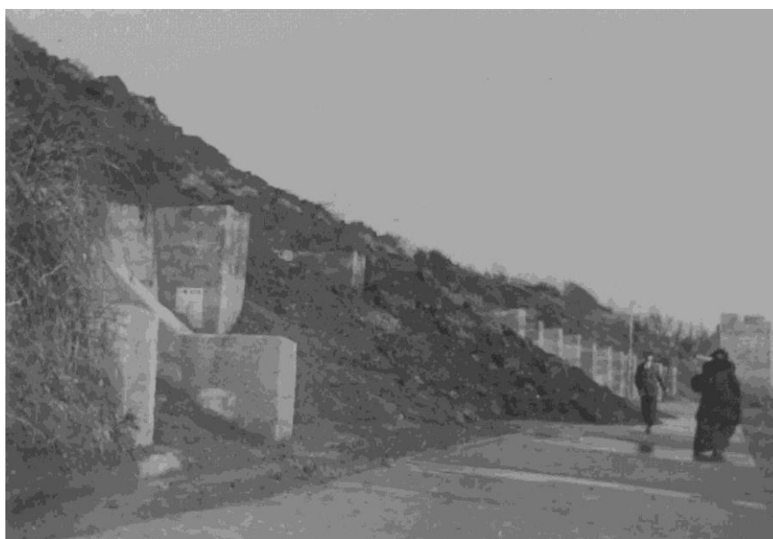
The 1903 buttresses being overwhelmed by landslip in 1925.
