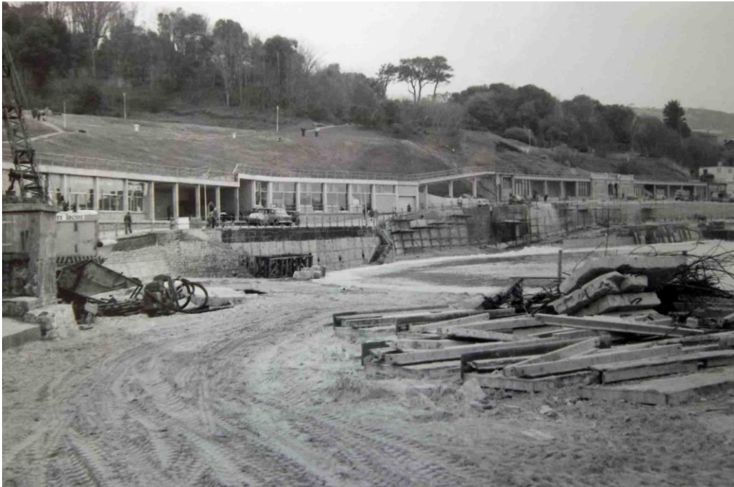
Marine Parade – the new Cart Road (far right) and Marine Parade walls being built in 1978-9. Note the two sets of shelters with the linking footbridge, and landslip resting on the roofs of the shelters to the right. The western shelters are fairly new in this picture.
