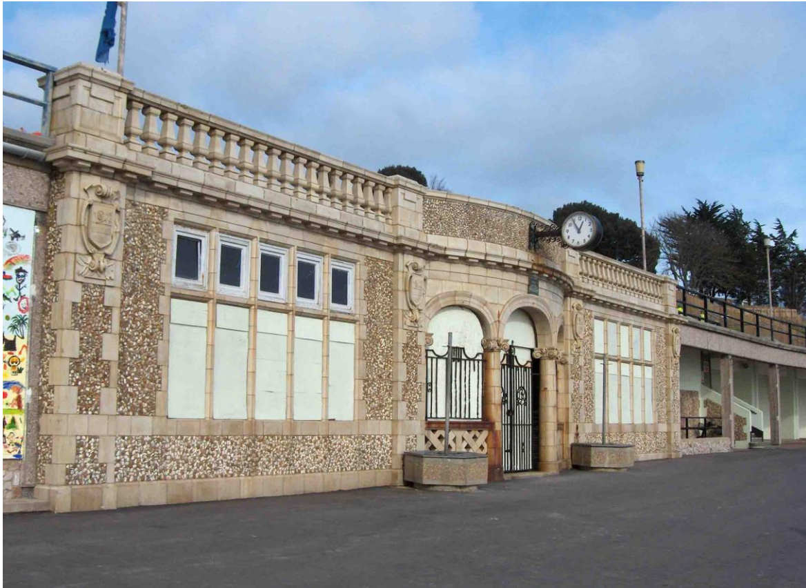
The Corporation Shelter and Eastern Open Shelters in November 2006, before refurbishment. The central pavilion is closed, but the roof is accessible again, now cleared of mud. It was restored as the Jubilee Pavilion. Through the shelters can be seen the 1903 concrete buttresses holding up the slope, painted pale greenish-blue.
