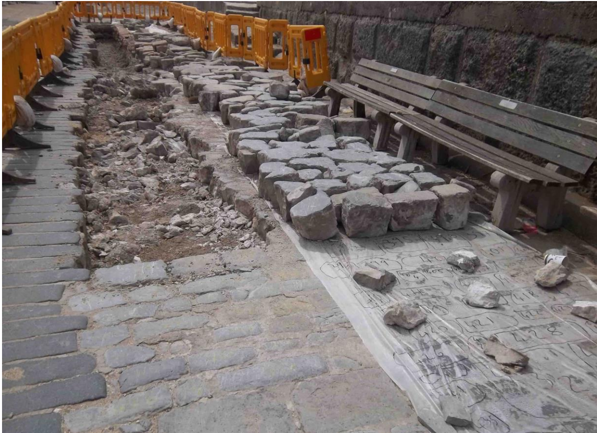
Replacing roadway cobbles in 2014 using a full-scale tracing for guidance
