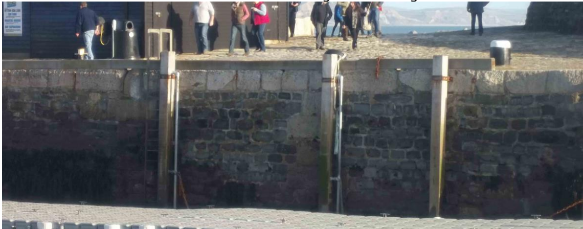
Extension to Landing Quayside 1829
