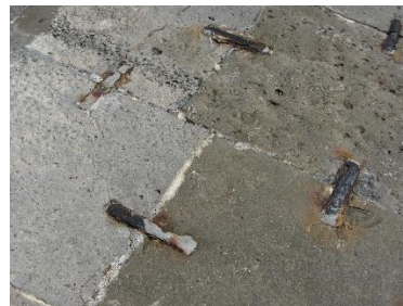
Iron Cramps on the Southern Arm
