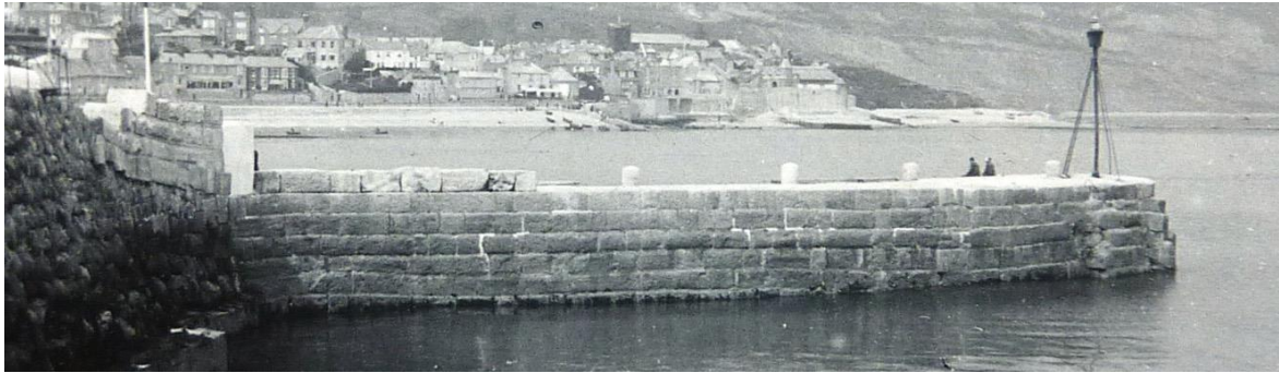
Victoria Pier in 1926 showing early signs of settlement. The pier abuts the termination at Crab Head by the white gents' loo. The loose Roach blocks still sit on the edge of the Pier, as do the sloping blocks on Crab Head. LRM Cobb Photo Box
