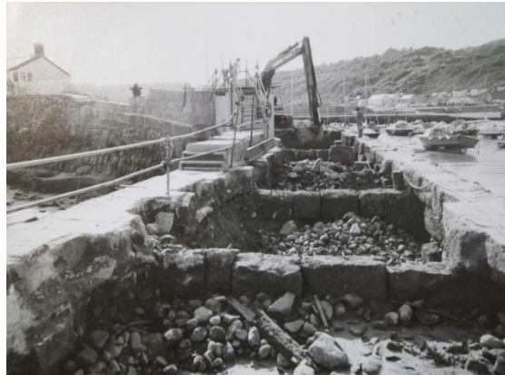
Original Hearting of Victoria Pier of 1842-8
