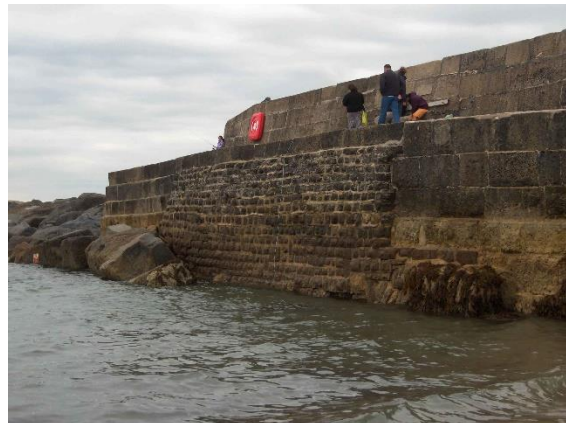
Three styles of construction, Left Surviving 1650s vertical Cowstone work butted to, and under, post 1817 Portland ashlar blockwork inside the High Wall at the Roundabout. Right Surviving Biscuit Work of 1762-3 below the walkway of the Southern Arm - horizontally laid squared Cowstone under Portland copings keyed and butted to the 1785 Portland ashlar tip of the Southern Arm, keyed and butted to 1795 Portland ashlar to the right.
