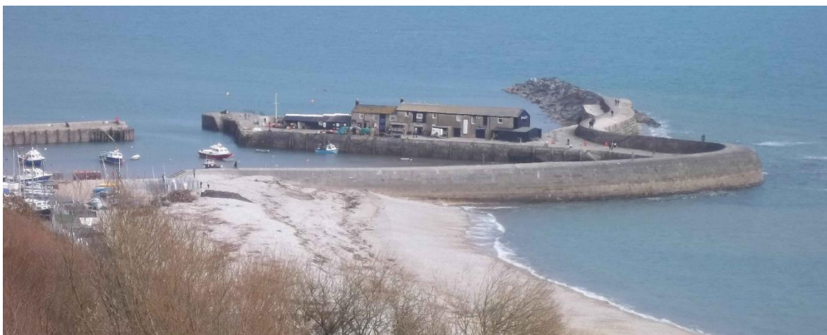
The curving High Wall of Lyme's principal breakwater up Monmouth Beach
