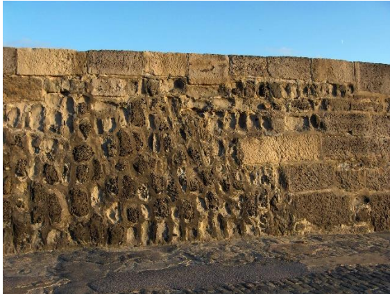
Three styles of construction, Left Surviving 1650s vertical Cowstone work butted to, and under, post 1817 Portland ashlar blockwork inside the High Wall at the Roundabout. Right Surviving Biscuit Work of 1762-3 below the walkway of the Southern Arm - horizontally laid squared Cowstone under Portland copings keyed and butted to the 1785 Portland ashlar tip of the Southern Arm, keyed and butted to 1795 Portland ashlar to the right.
