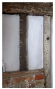
front wall to accommodate a fireplace in the adjoining room and most likely of the late 18<sup>th</sup>, early 19<sup>th</sup> C. Further along the hall the top support beam of the plank structure has been crudely chopped through [right] to insert a door way
