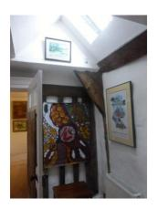
On the west partition, there is plank & muntin walling [above left], this aligns with the wall on the lower floor and the cruck frames and would support the idea that they are original and in situ. As in the passage downstairs they have been altered, the original upper and lower horizontal frames are in situ with some of
